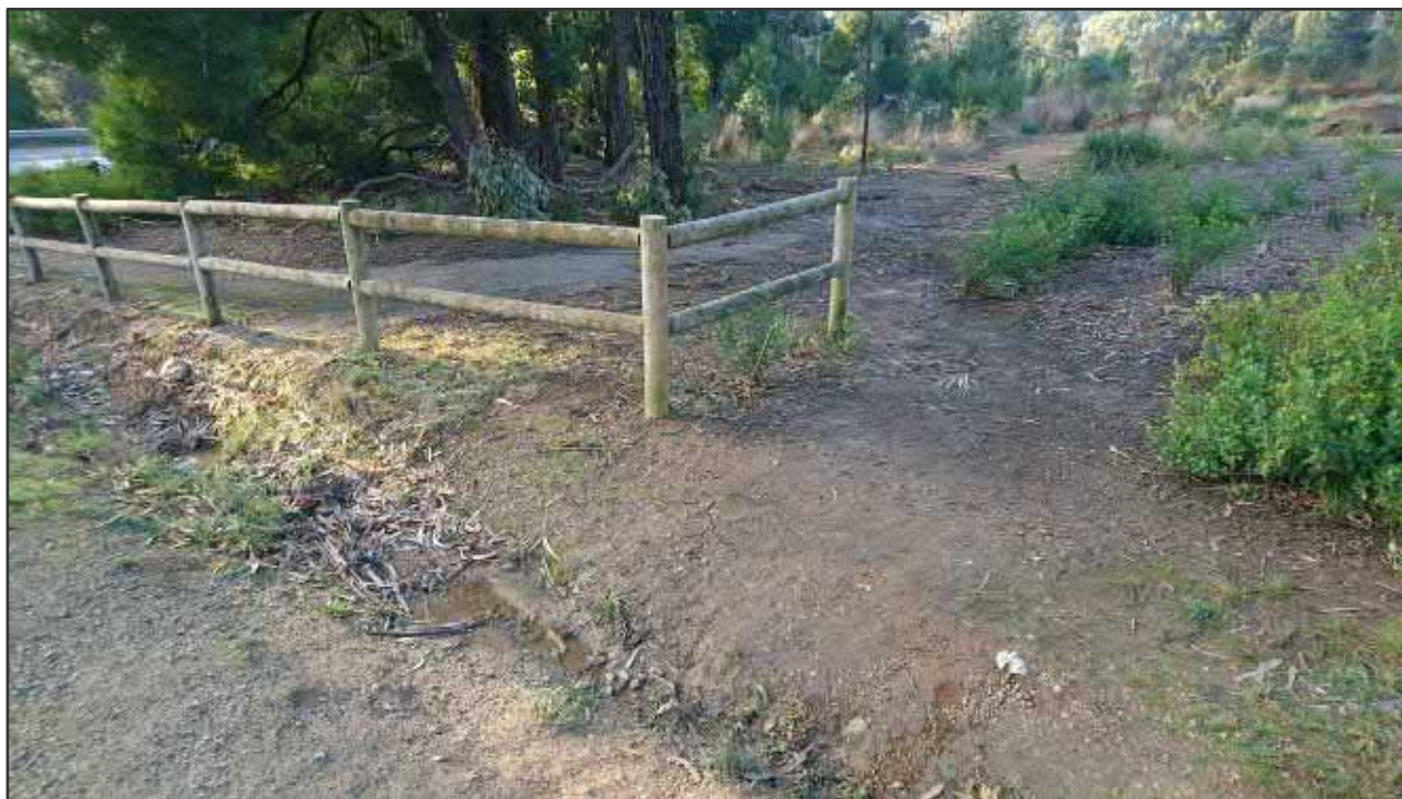
Figure 65 Bypass of the Pedestrian Crossing on Point Leo Road
