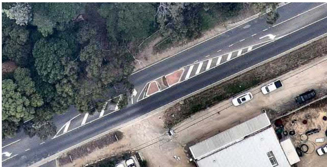
Figure 66 Existing Pedestrian Crossing – Shoreham Road
