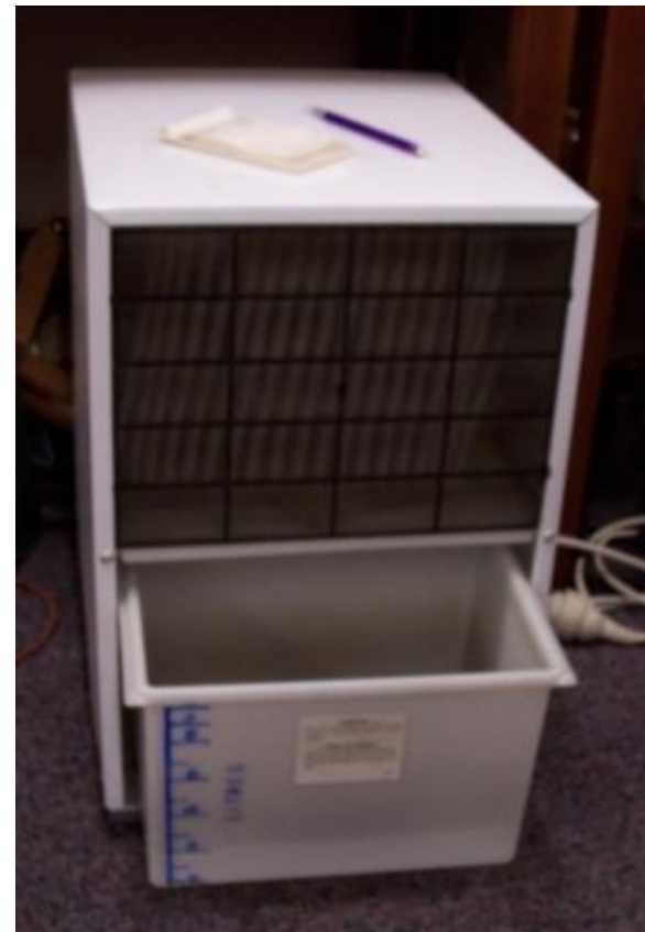
Figure 18: Dehumidifier runs 24/7 to extract excessive humidity from display room
