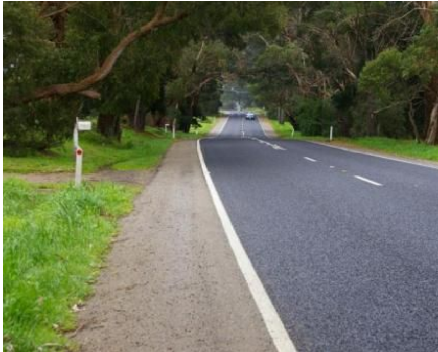
Figure 4.22 Browns Rd sealed shoulders should be bicycle lanes and appropriately marked
