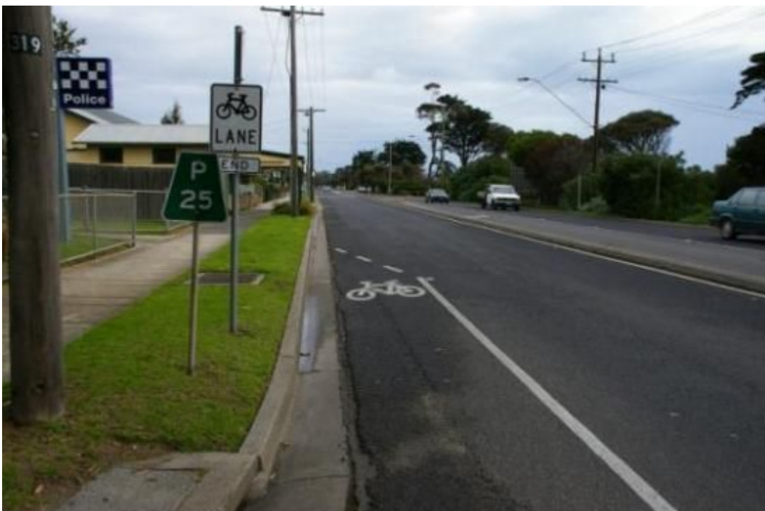
Figure 3.2 Bicycle Lane continuity is important along Point Nepean Road
