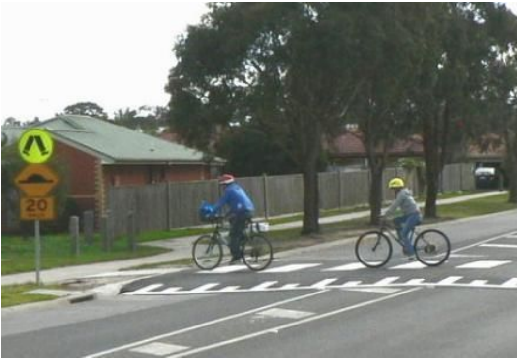
Figure 4.16 New raised speed hump and pedestrian crossing Bentons Road
