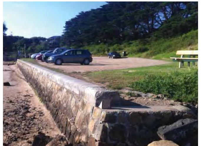
Stone sea wall at the outlet of Tanti Creek. The western carpark is used by visitors to view the water from their vehicle.
