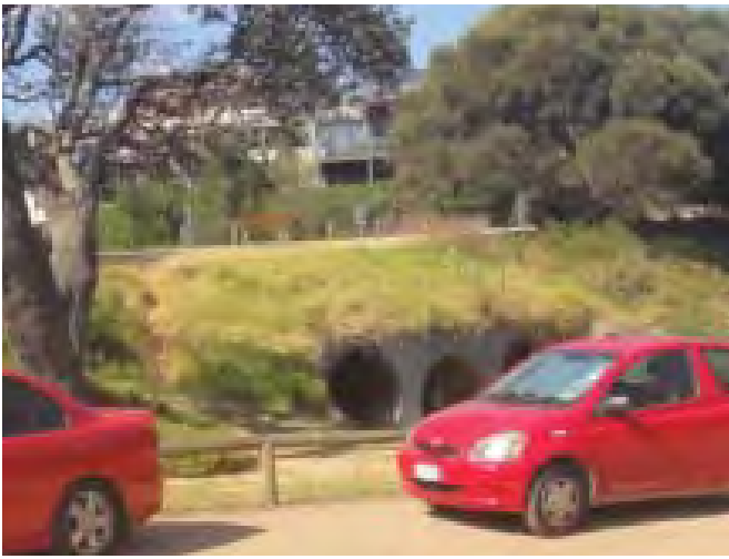
Stormwater pipe beneath the Esplanade. Opportunity for revegetation and improved pedestrian facilities.
