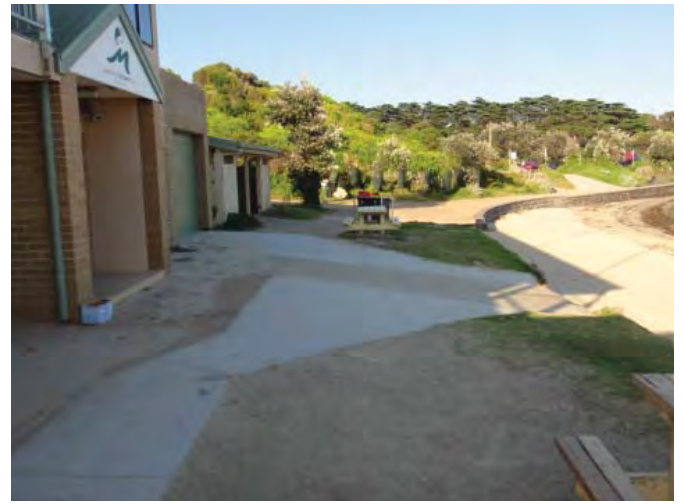
Existing ramp to front of LSC very steep for deployment of rescue boat. The ramp can become slippery when covered in sand.
