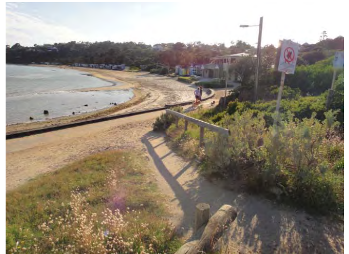
Access to the beach and LSC is narrow, steep and only partially sealed, making access difficult for some people with limited mobility. There is an opportunity to improve access to areas and cater better for people of all abilities.
