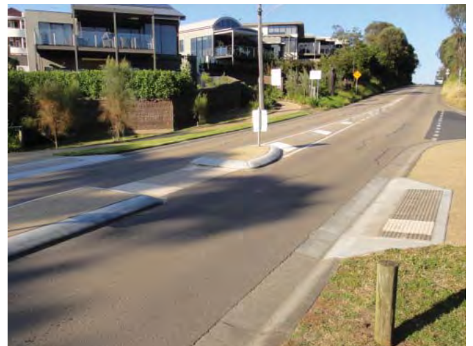
Recently installed pedestrian crossing creating a pedestrian connection to the surrounding residential areas.
