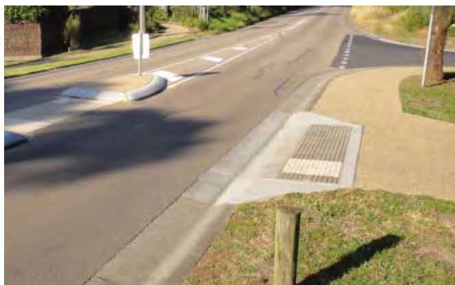
Figure 5.1 Existing exposed aggregate footpath and crossing on the Esplanade at Mills Beach
