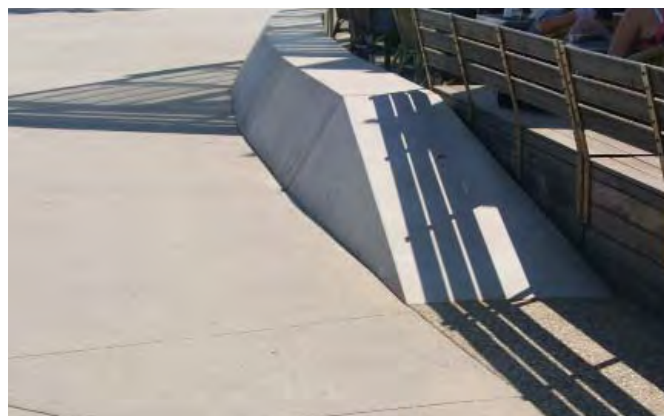
Figure 5.4 Example of a concrete retaining/seating wall in exposed aggregate concrete at St Kilda Baths
