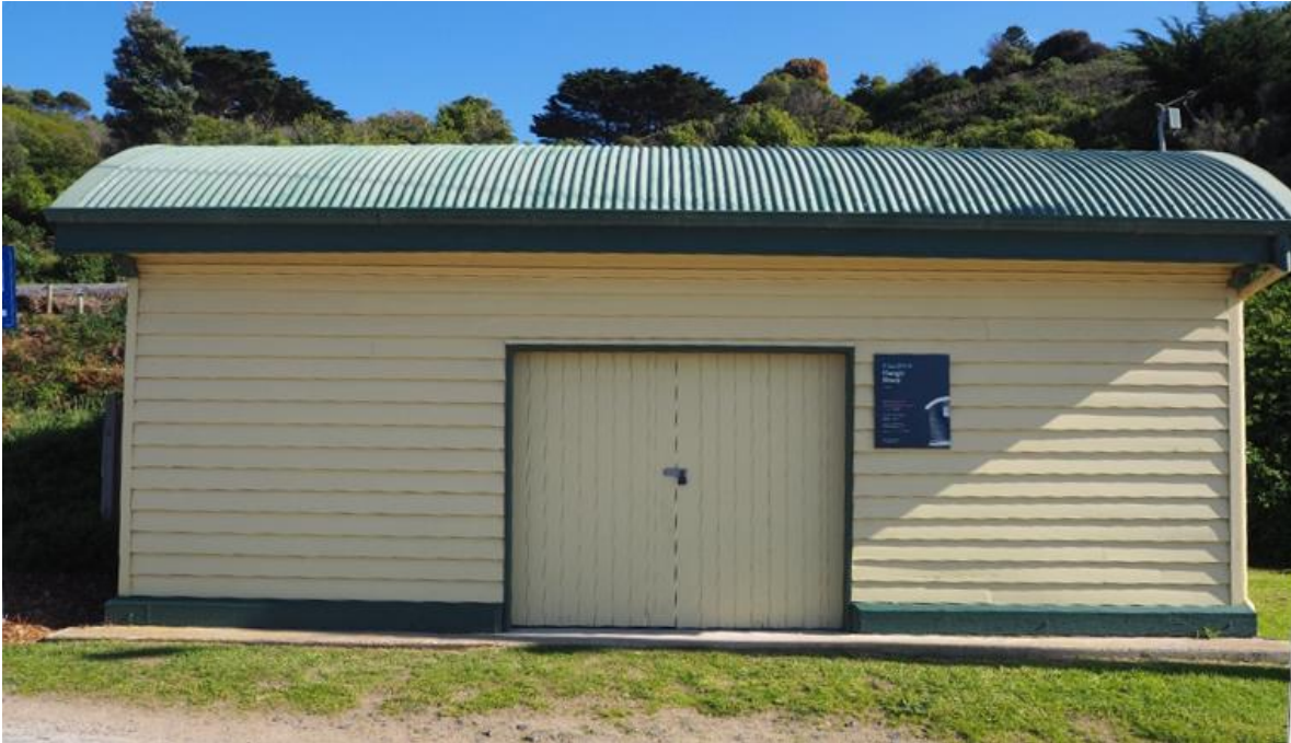
Figure 53: 1871 Cargo Shed following restoration (G. Vines 2023)
