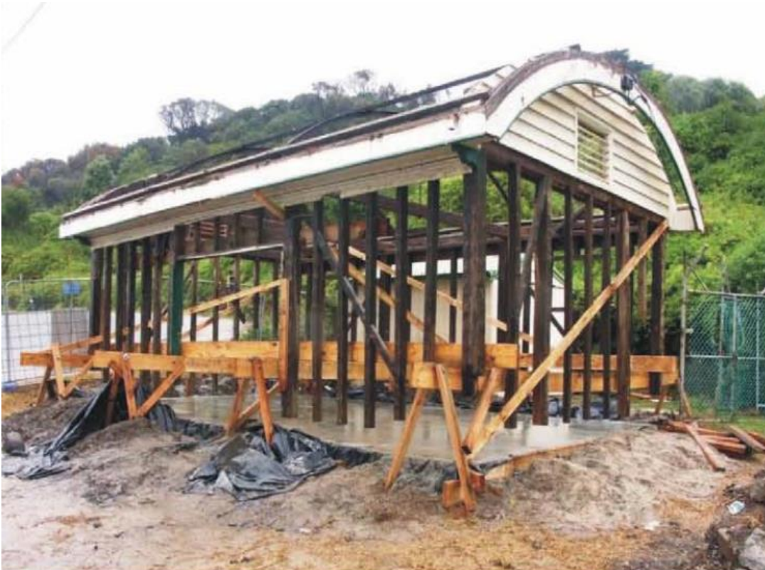
Figure 79: Cargo shed during restoration showing new concrete floor slab and wall studs cut at base for scarfing
