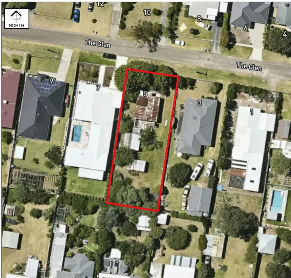
Figure 1. Aerial MetroMap image dated 29 December 2025.
