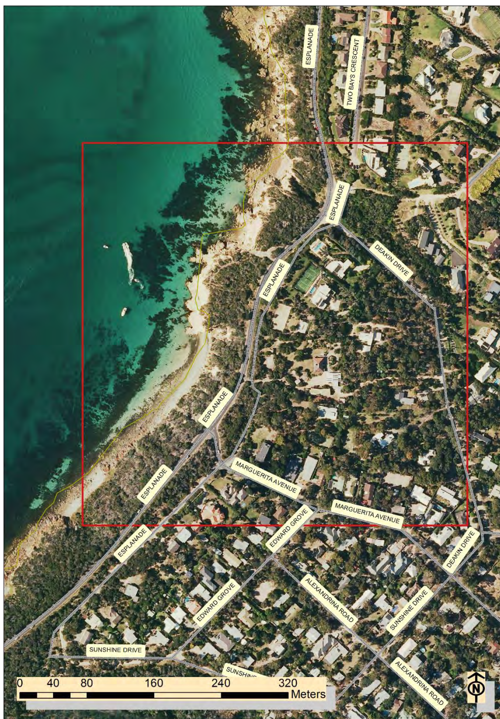
Figure 2 - Aerial view of 'Pillars' assessment area
