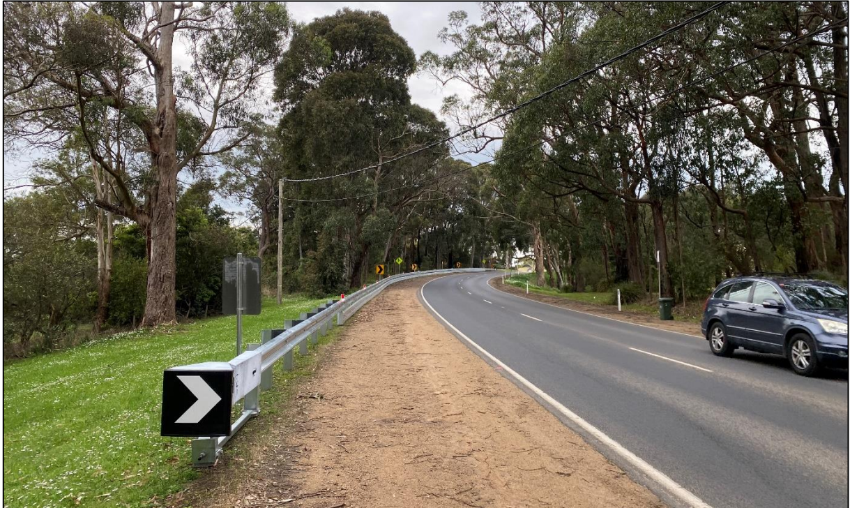
Photo 1: Arthurs Seat Road approximately 200m east of White Hill Road, facing east
