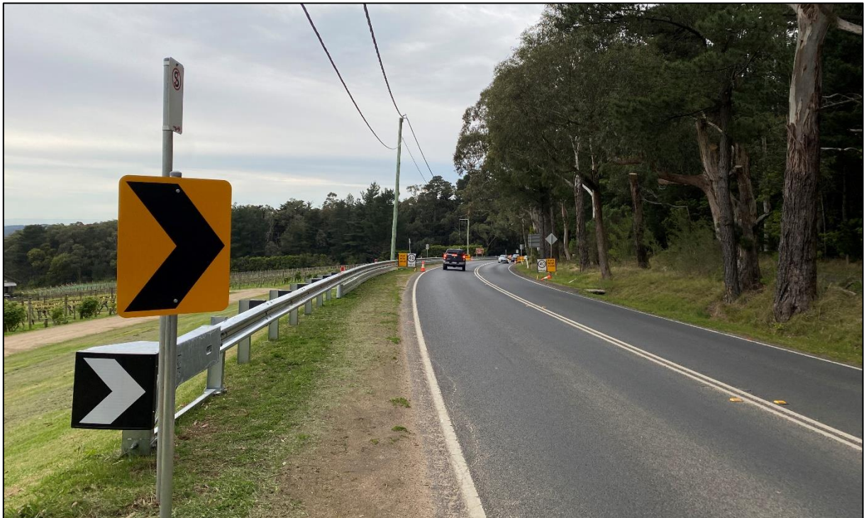
Photo 5: Arthurs Seat Road adjacent Eldridge Estate, facing east
