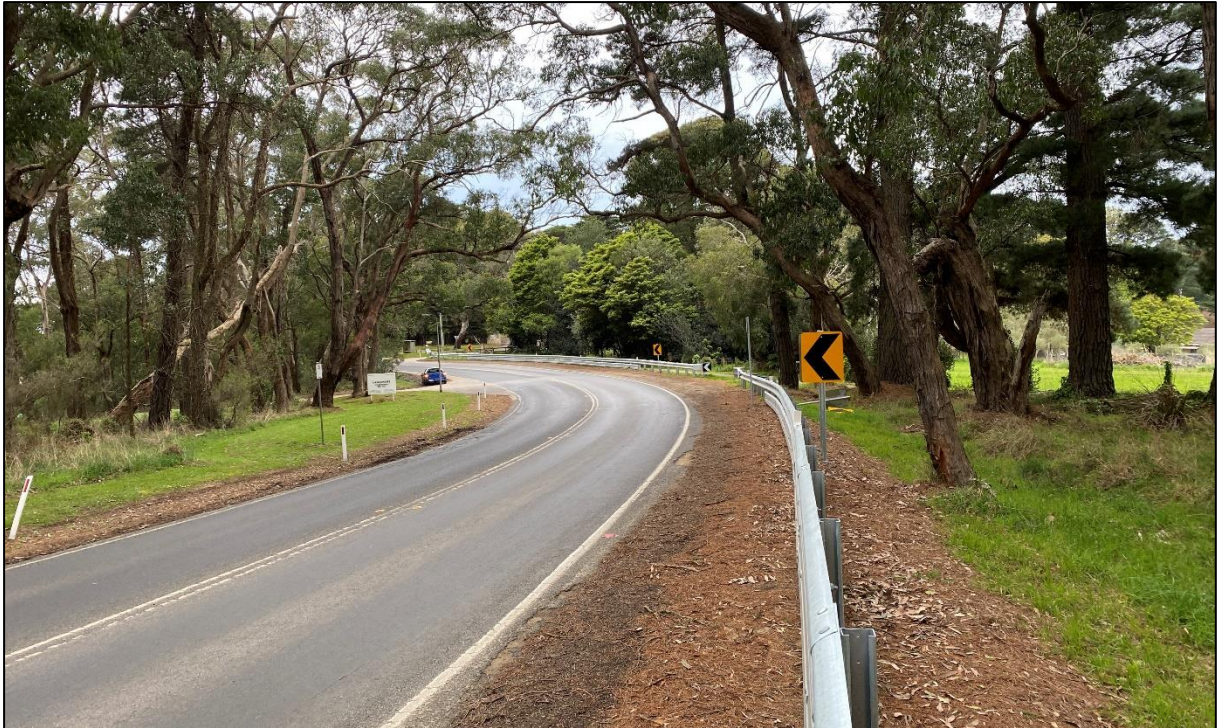
Photo 3: Arthurs Seat Road near Andrews Lane, facing east
