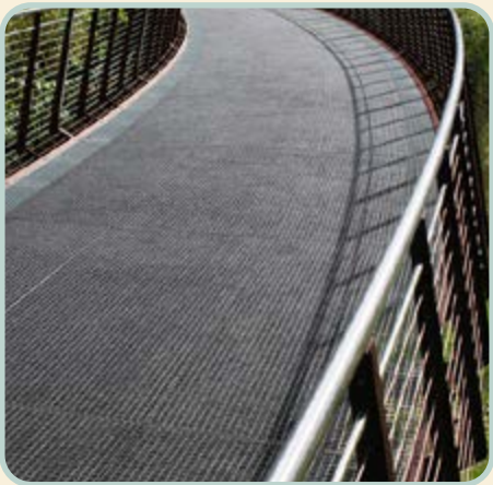
Fibre reinforced plastic (FRP) boardwalks
